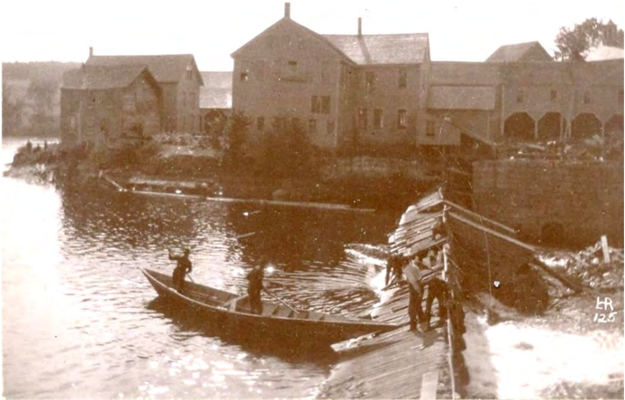
Figure 14. Pre-1883 photo showing the wood planking being replaced on the upstream face of the dam. Source: Dover-Foxcroft Historical Society.
