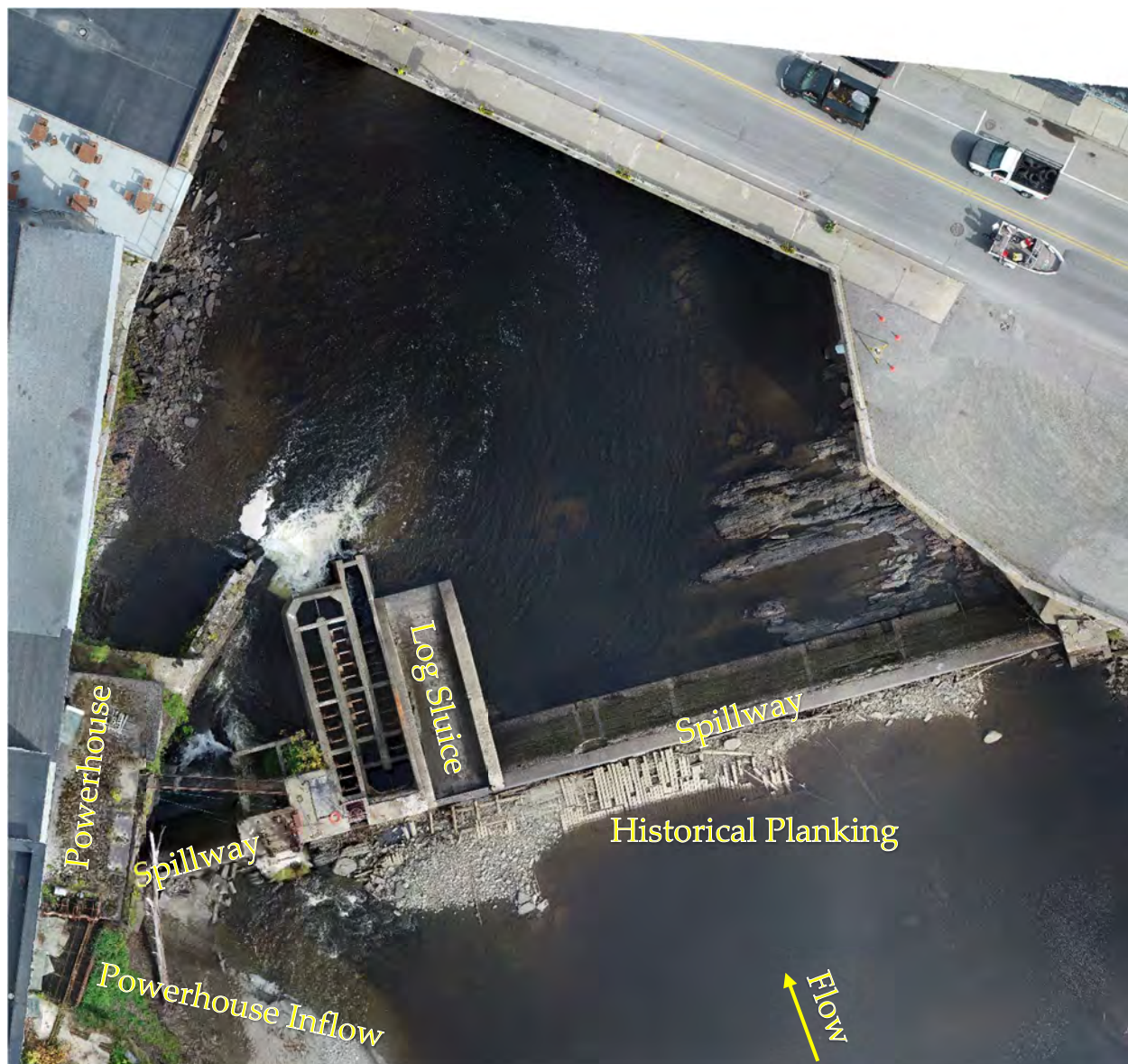
Figure 26. September 2019 aerial photo during drawdown showing features of the dam. Source: Webber Surveying.
