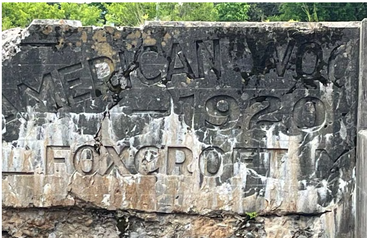
Figure 23. 1920 inscription in 2022, modified in 1982 with construction of the Denil fishway.
