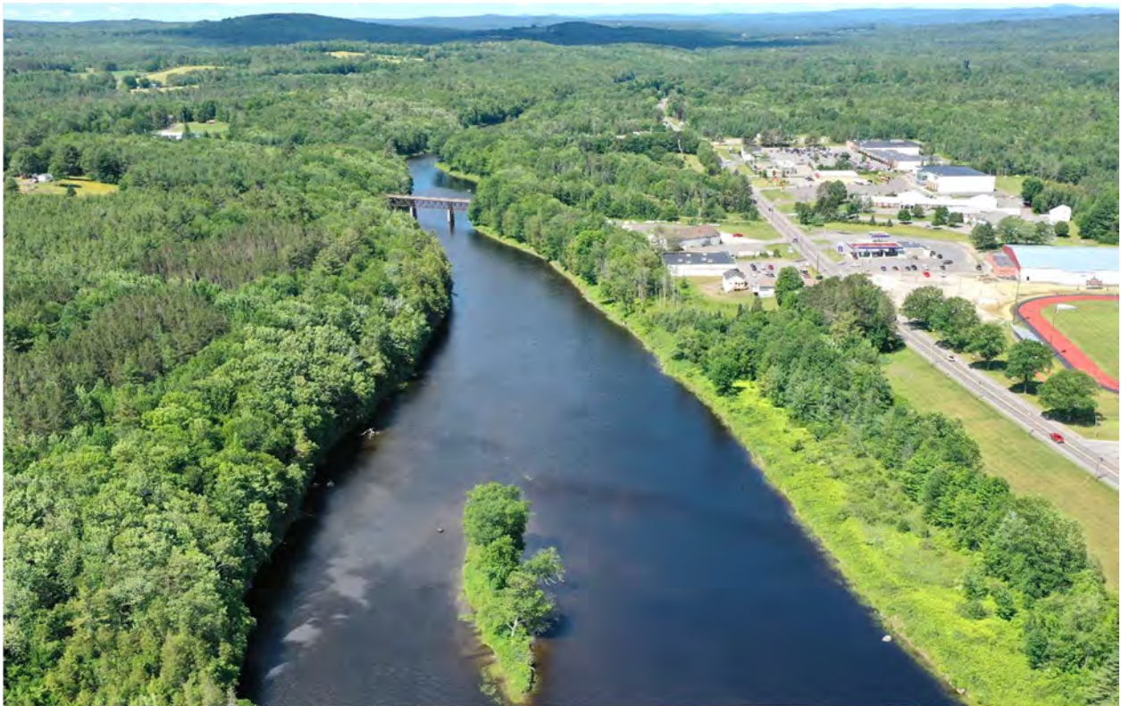
Figure 43. June 2022 view looking upstream at impoundment Zone 4.
