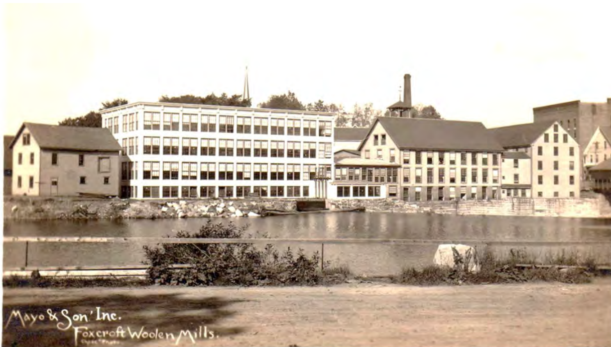
Figure 5. Image showing the original two mill buildings, and the first concrete structure constructed in 1908. Source: Dover-Foxcroft Historical Society.
