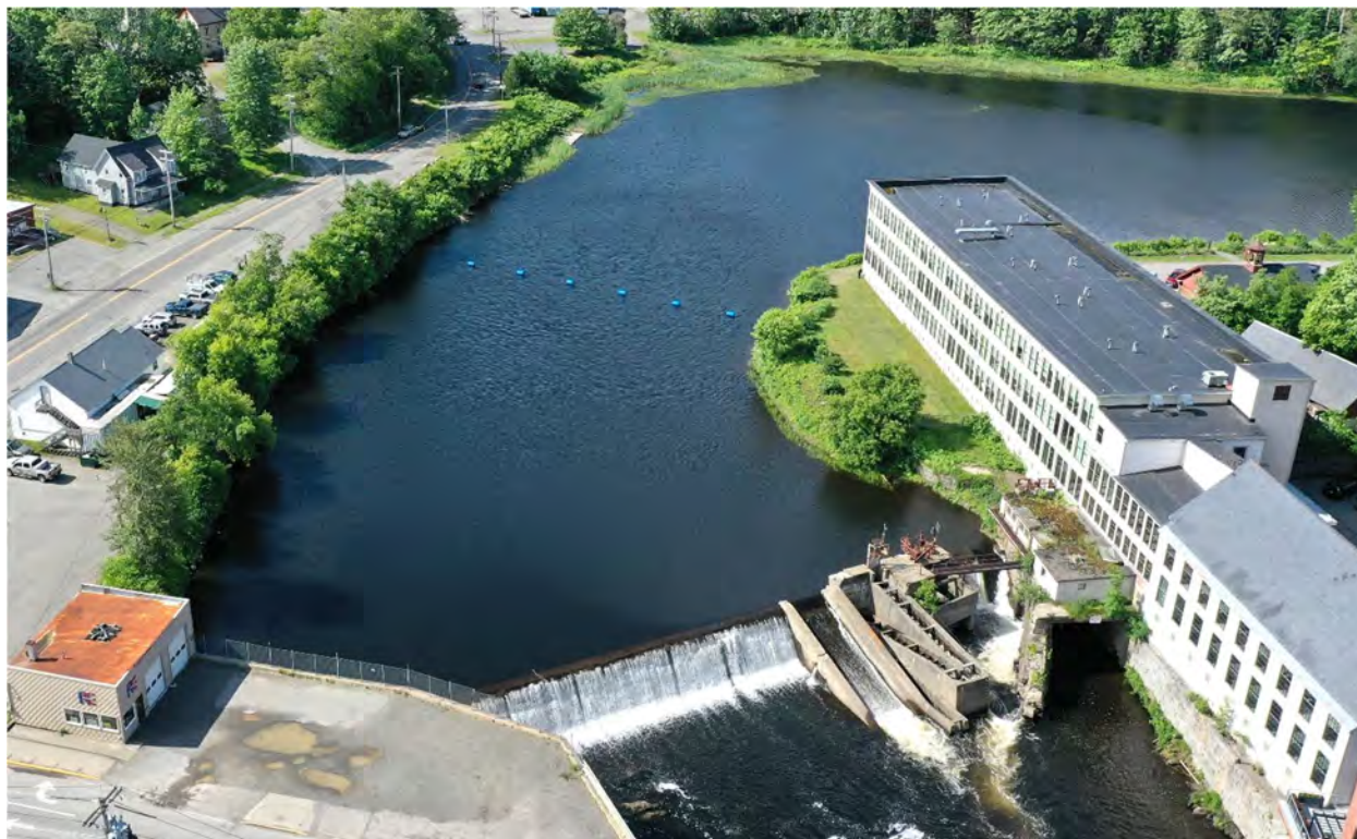
Figure 38. June 2022 view looking upstream at impoundment Zone 1.
