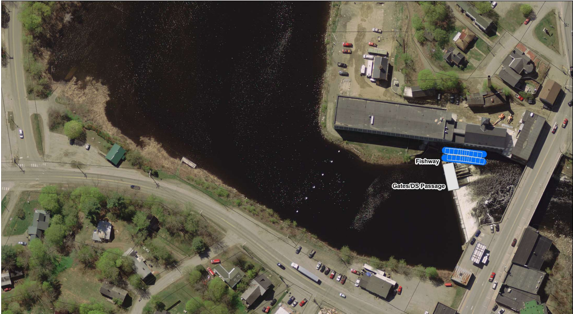
Figure 2. General location sketch for options F 1 and F 2 (Retain Dam, Maintain Impoundment at Current Levels, Technical Fishways, FERC Exemption Retired), and L 1 and L 2 (Modify Dam, Retain Impoundment at Lower Level, Technical Fishways, FERC Exemption Retired). Actual configuration, orientation, scale and size will vary pending additional development.
