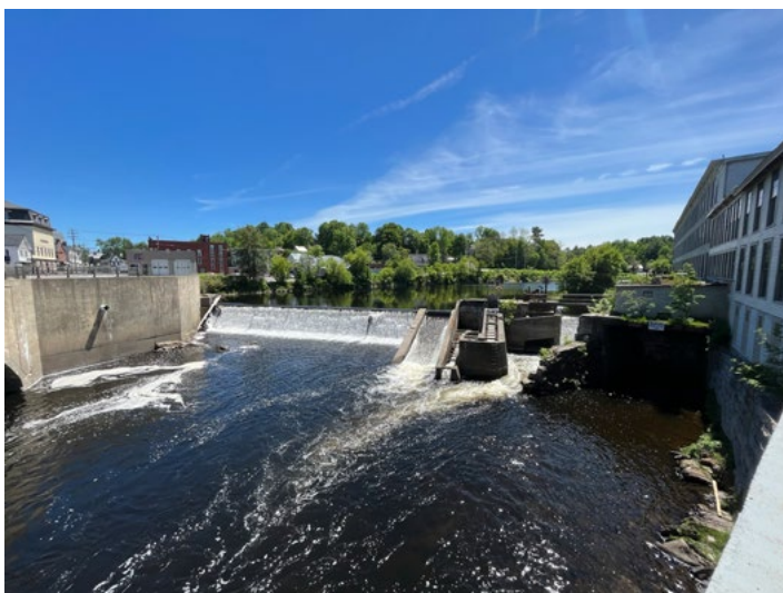
The dam site in 2022.
