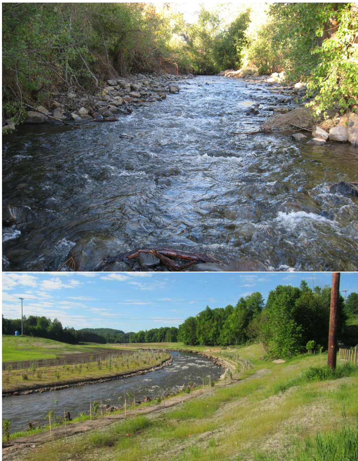
Figure 13. Examples of constructed nature-like fish passage. This type of fishway is considered under Alternatives N6 and N7.
