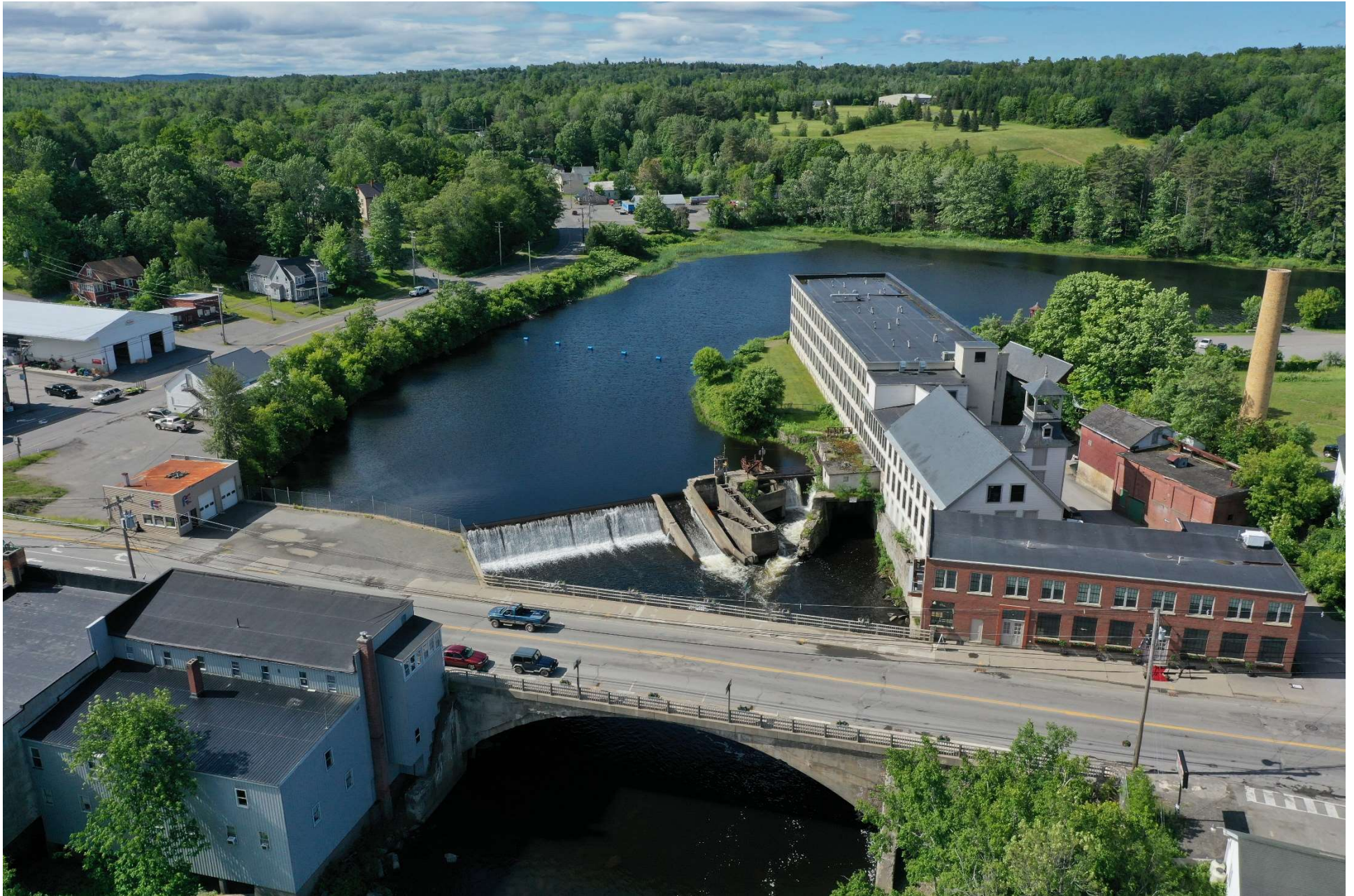
Figure C-1. Existing condition looking upstream at Mayo Mill Dam, June 20, 2022.
